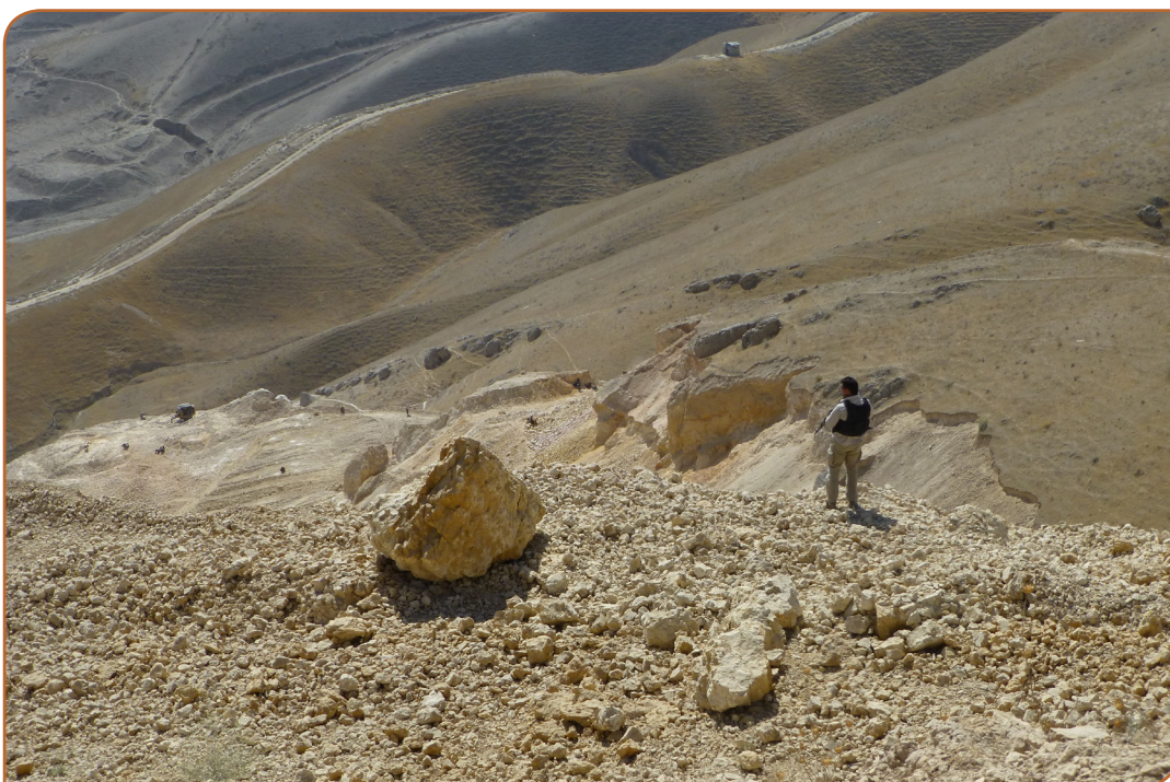
Left - Figure 2: The Ghorl I plant is located between an 87Mt limestone hill and the Pol-e-Khomri River. The hill and river provide a significant portion of the plant's raw materials.
