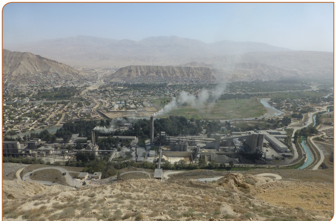
Right - Figure 1: The Ghorl I cement plant was commissioned in 1959 by the Afghan Government. It is some 200km North of the capital city, Kabul, near the Pol-e-Khomri District, Baghlan Province.
